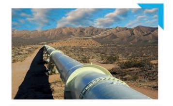
The polyurethane insulation used in our insulated oil pipes guarantees not only excellent thermal insulation but also mechanical protection. High oil temperatures are easily maintained in our pre-insulated oil pipes and the oil remains at a constant viscosity, meaning it can be pumped with greater energy and cost efficiency.
