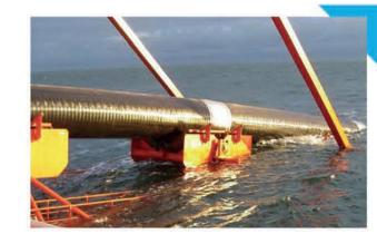
Ecoline has developed a pre-insulated solution for the large diameter loading lines for onshore LNG-terminals, eliminating any maintenance that traditionally insulated lines require over the service life of a project. The entire system is completely water- and airtight.
